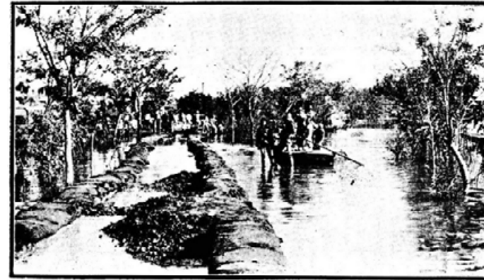
FILLING DYKE WITH MUD FROM BOATS.
